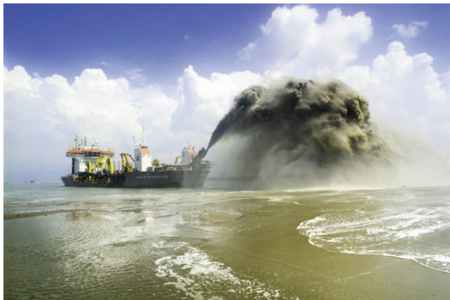
Figure 2 | 'Building with nature'. Beach nourishment is one alternative approach to engineering in flood management along the Dutch coast.
